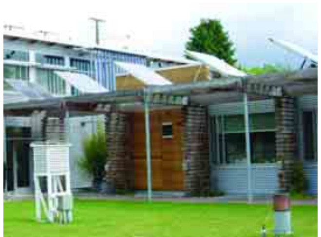
Exhibit 4.31 Green Operations Building: photovoltaic array
