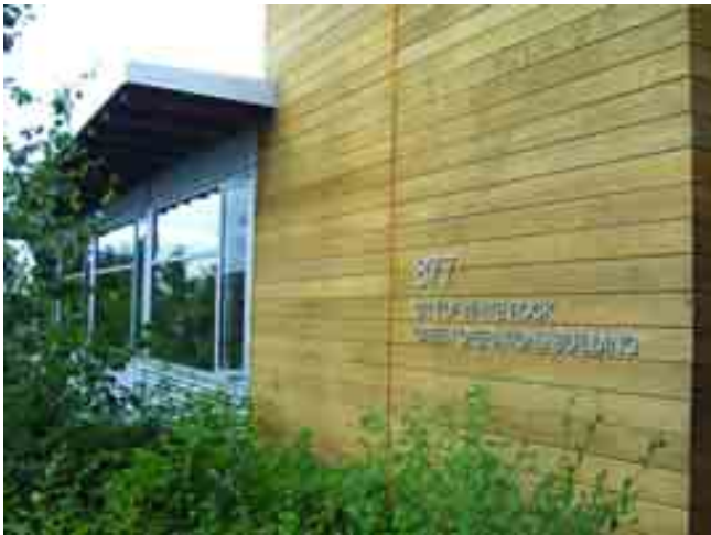
Exhibit 4.26 City of White Rock, BC, Green Operations Building
