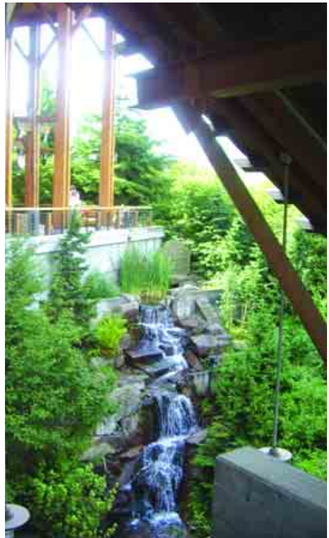
Exhibit 4.40 REI flagship store: building and nature
