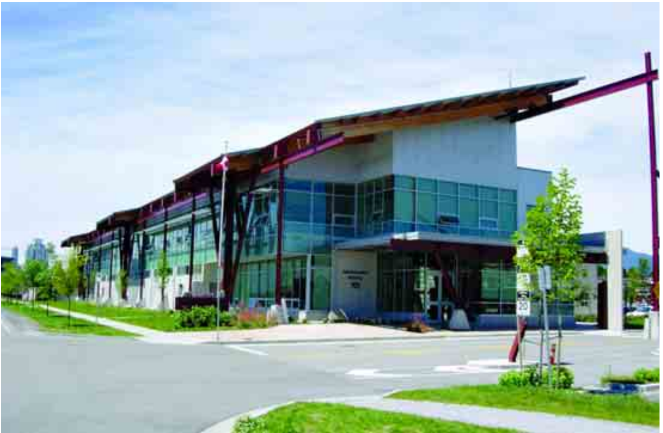
Exhibit 4.3 City of Vancouver Works Yard
