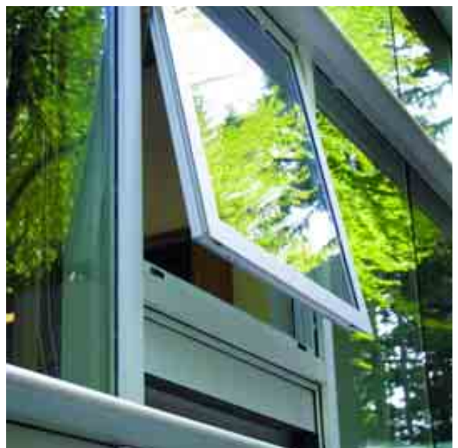
Exhibit 4.13 Liu Centre: operable windows
