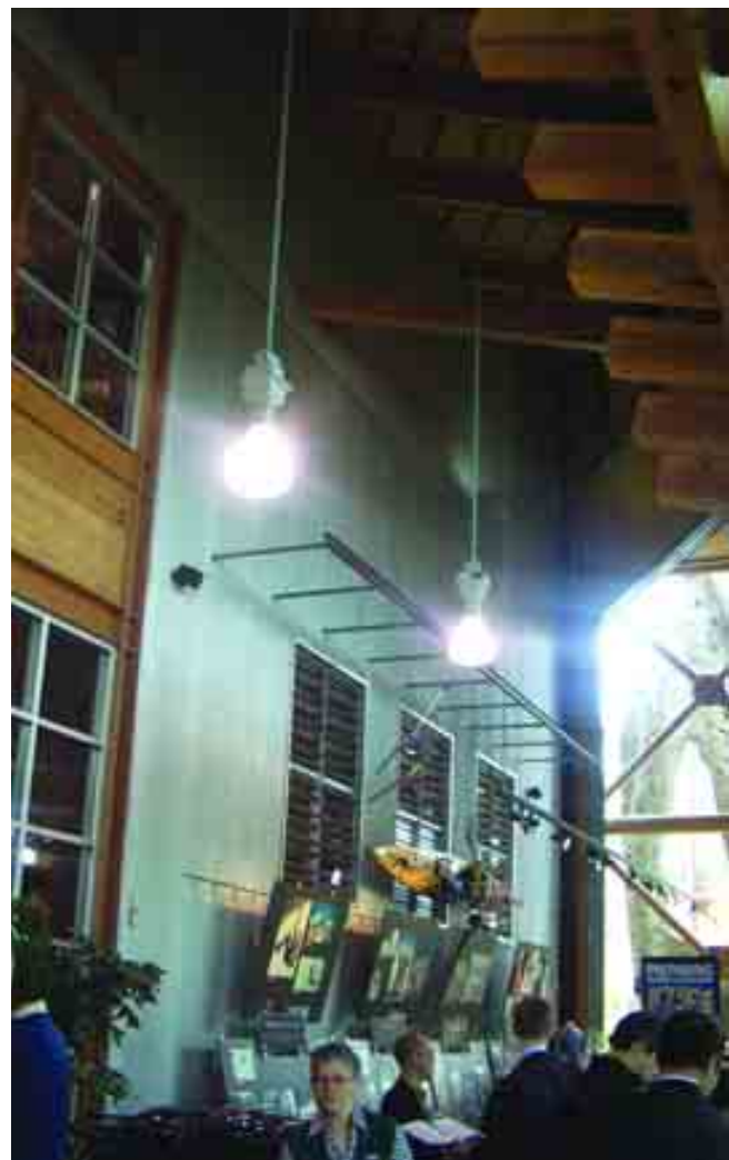
Exhibit 4.44 REI flagship store: automatic dampers control natural ventilation paths
