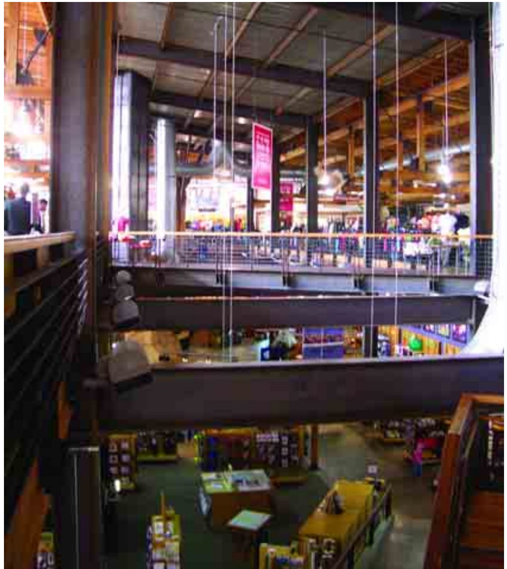
REI flagship store: steel and timber construction
