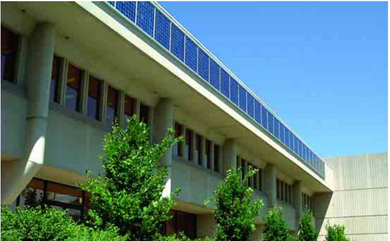
Exhibit 2.11 Photovoltaics at UTM
