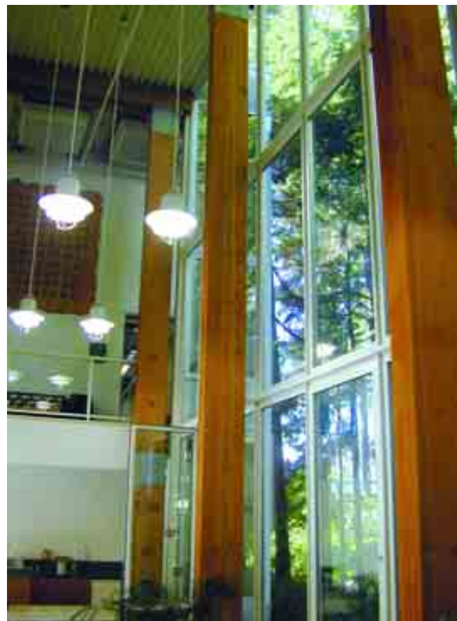
Exhibit 4.8 C K Choi Building: atrium on western flank
