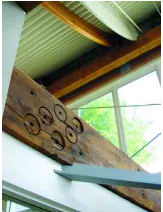
Exhibit 4.9 C K Choi Building: recycled timber bearing scars
